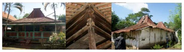
Omah dudur loro exterior (left and right figure). Insen/tumpang construction in omah dudur interior (center figure)
